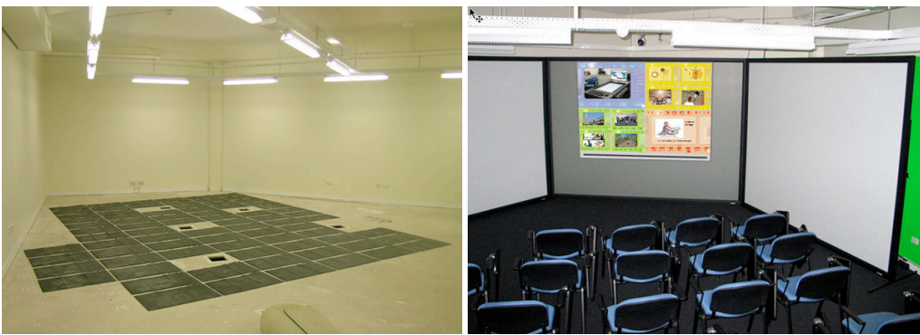
Figure 4: The pressure sensitive pads placed underneath the carpet (L), “The Sentient” with completed flooring (R)
